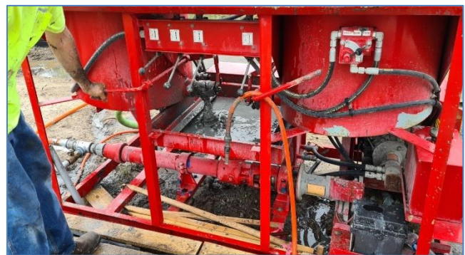
Figure 21 – Grouting mud being mixed and discharged into the pump chamber.
