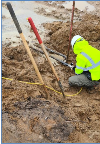
Figure 14 – Pressurizing a completed loop
