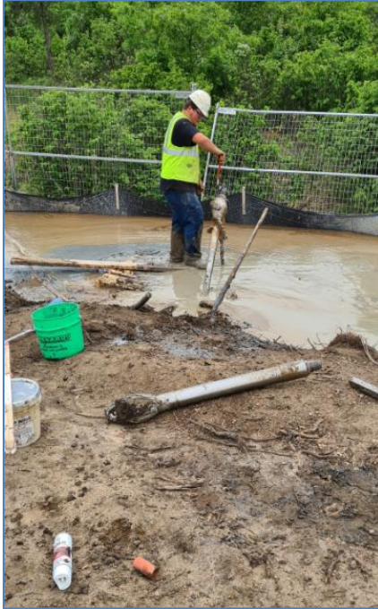
Figure 11 – Preparing back-reamer for pulling the loop into the borehole
