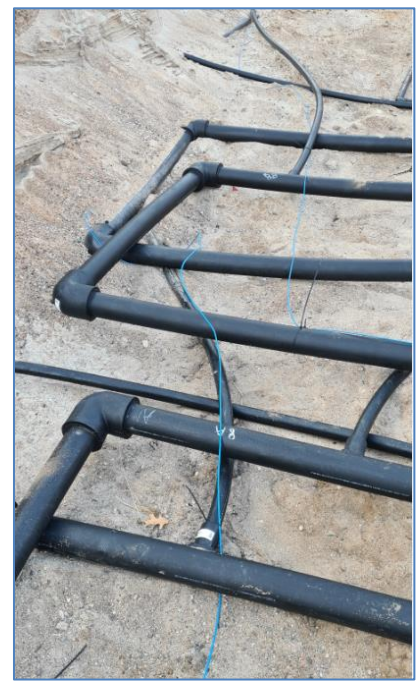
Figure 46 – Circuits at E Wall of Trench where the Connections Reverse
