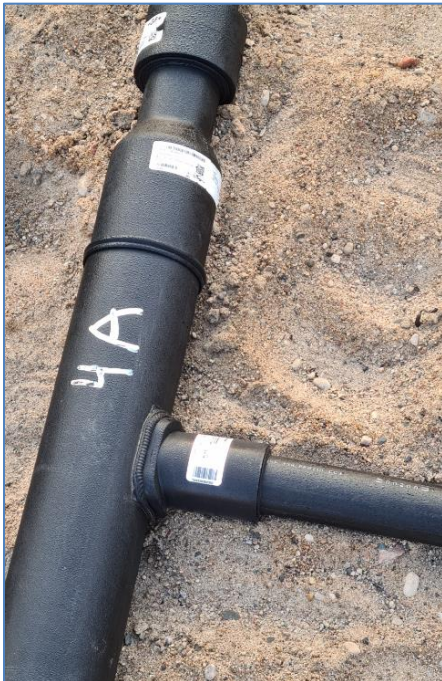
Figure 44 – Typical Saddle Fusion and Circuit Markings
