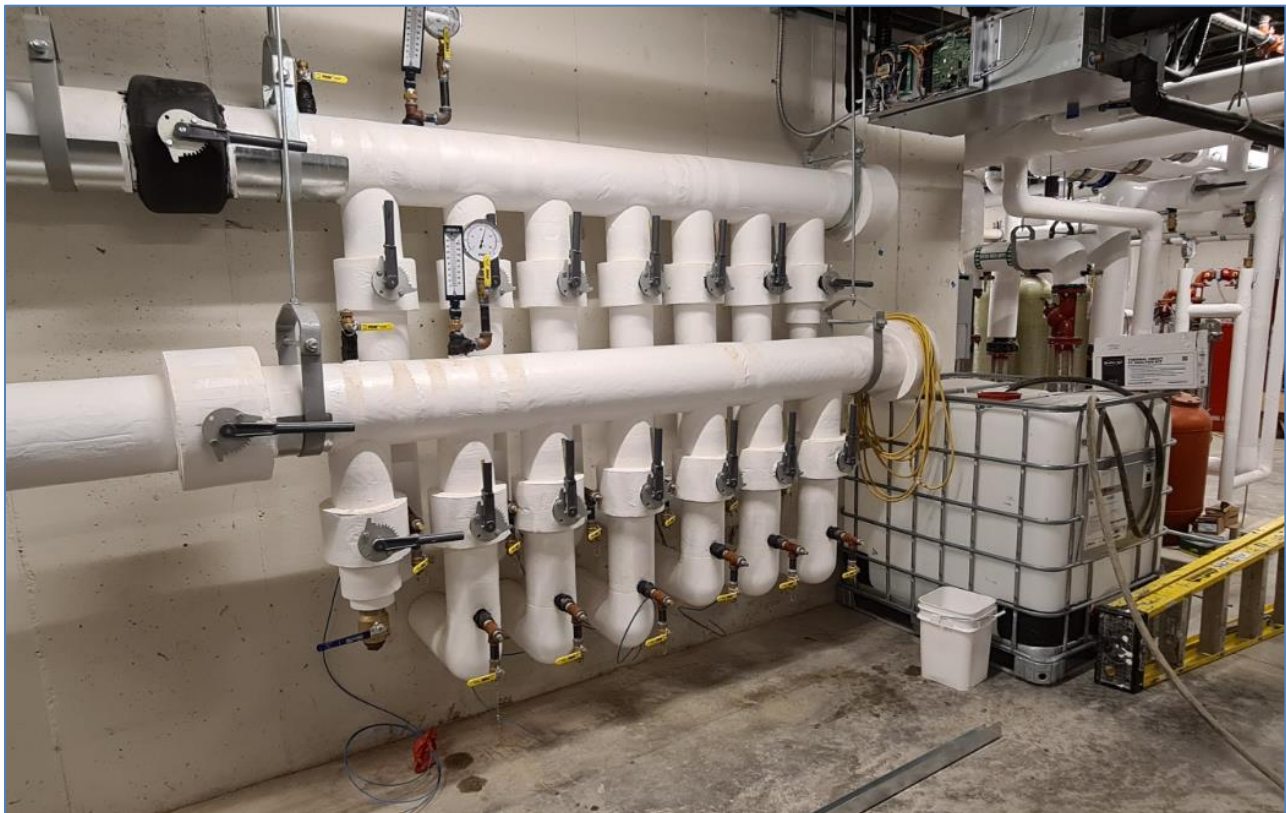
Figure 68 – Mechanical area with GHX Circuits and Final Valve Positions. The Tote to the right is for the 55-gallon supply of Glycol Solution to be left for future use as needed. It is the 30% field mix that is used in the GHX.
