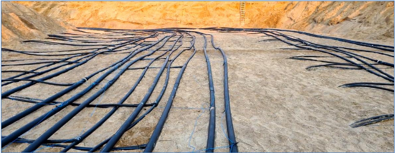
Figure 47 – Circuits and Tie-Ins ready for Pressure Testing
