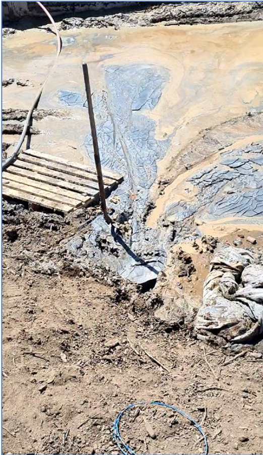
Figure 24 - Evidence of Graphite in Grout
