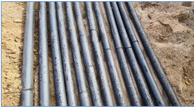
Figure 33 – Supply/Return Lines showing butt fusions
