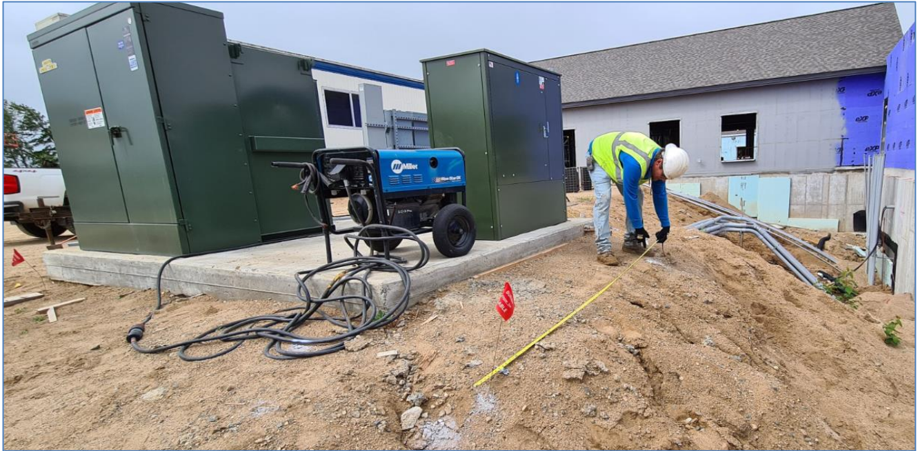
Figure 29 – Checking locations of loops that run beneath the electrical service hookups
