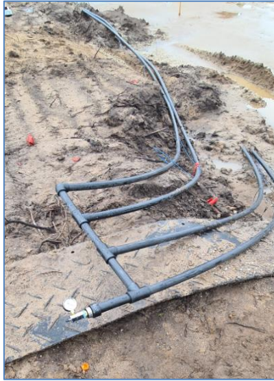
Figure 15 – Temporary manifold to pressure test more than one loop at a time.
