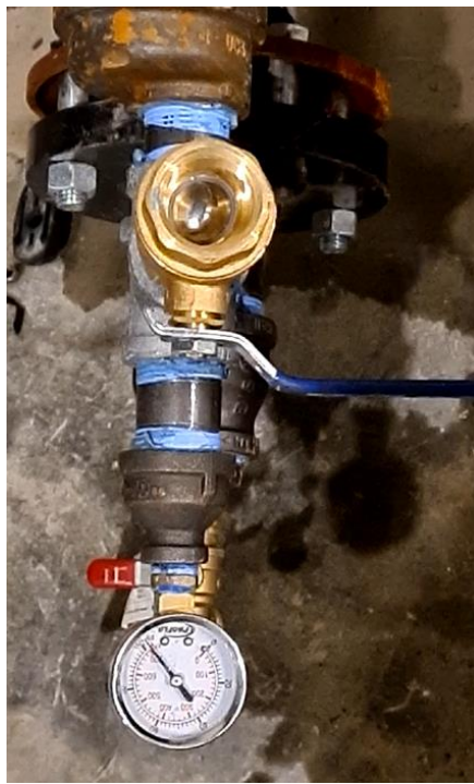
Figure 49 – Each Circuit (x6) Filled with Mains Water and Pressurized to 100PSI
