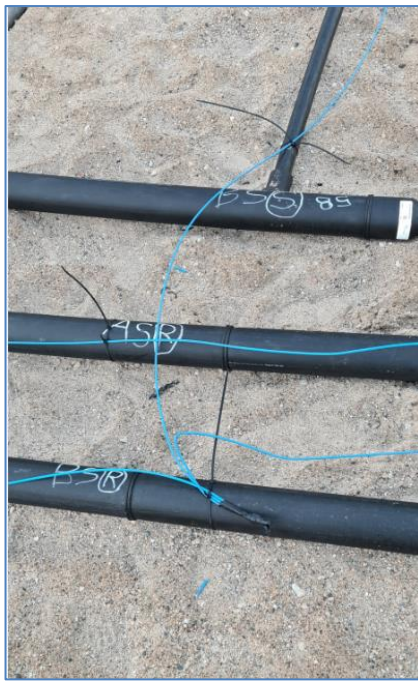
Figure 45 – Supply/Return Circuit Markings and Tracer Wires
