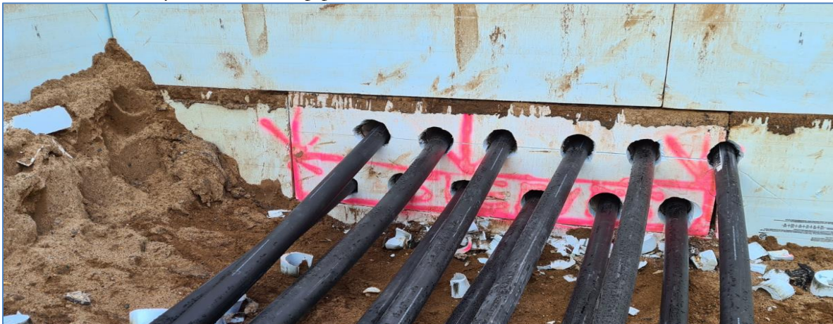
Figure 30 – HDPE supply/return lines from the loopfield to the Building Mechanical Room
