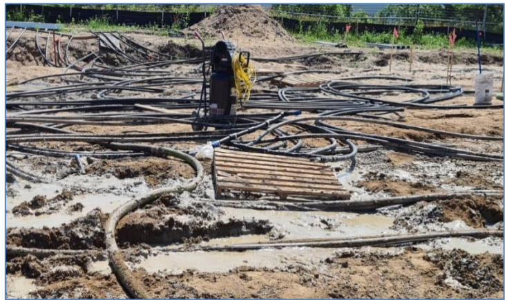
Figure 26 – The tailpieces of numerous installed loops
