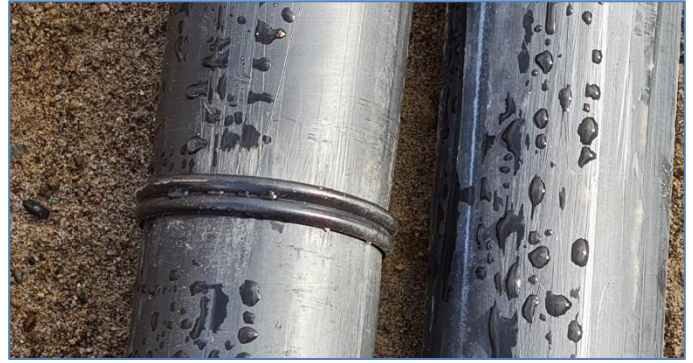
Figure 34 – Close-up of butt fusion of the 3" supply line
