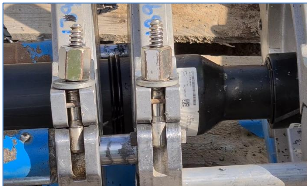
Figure 38 – 3" Butt fusion in process
