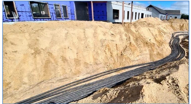
Figure 32 – Supply/Return trench and circuits across the front of the building
