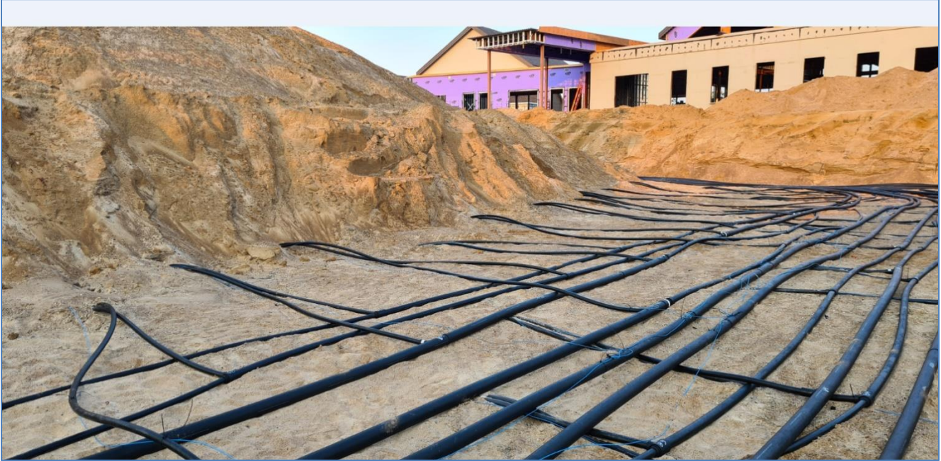
Figure 43 – Loop Tie-ins and reducing headers connected to the circuit piping. Pipes were hand bedded for separation prior the system being covered. Tracer wires showing and connected back to each circuit pipe into the mechanical room.
