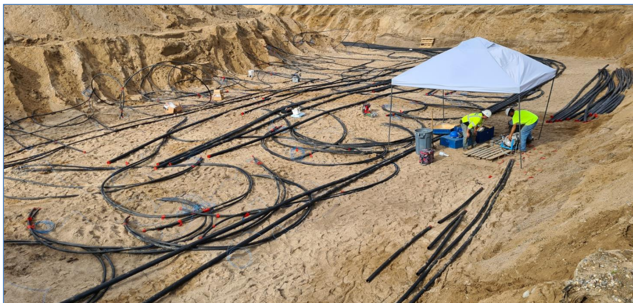
Figure 39 – Area excavated for circuit tie-ins to loopfield and working area for preparation of 3" circuit supply/return lines.
