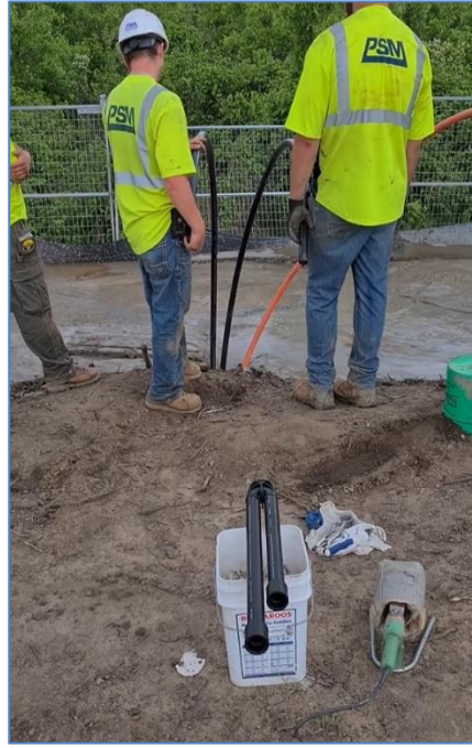
Figure 12 – Preparing the pipes to add the U-Bend to be pulled into the borehole
