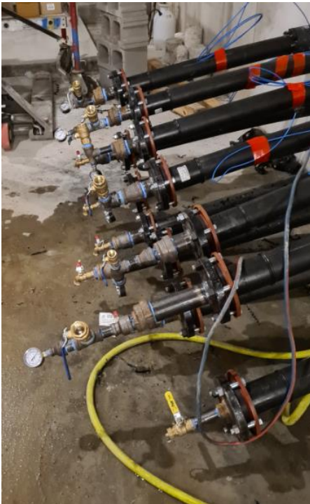
Figure 48 – All Circuit Pipes in Mechanical Room Temporarily Plumbed for Testing
