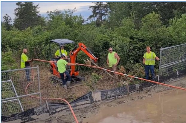
Figure 22 – When manpower was not enough to remove the tremie pipe
