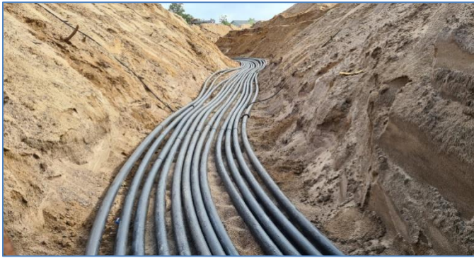
Figure 31 – Supply/Return run-outs from the Mechanical Room to the loopfield Tie-Ins
