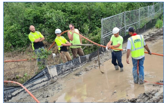
Figure 23 – Manpower was used to extract the tremie pipe as grout was pumped into the borehole
