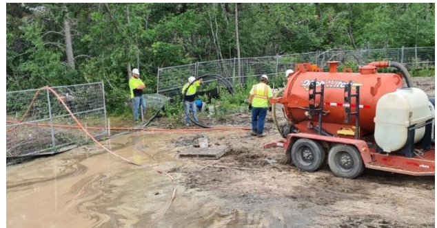
Figure 28 – Mud pumps used to manage grout and mud
