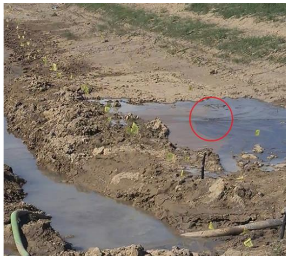
Figure 25 - Hydraulic Pressure Breakthrough on Pond Bottom. Note Evidence of Graphite in Grout.
