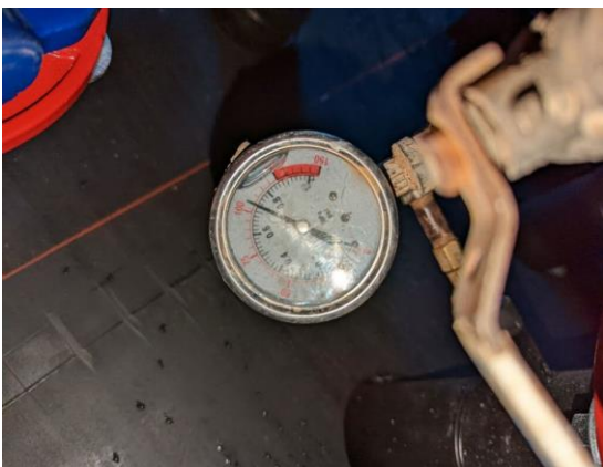
Figure 47 – Pressurized Circuit Under 24 Hour Test and Isolated in the Geothermal Vault.
