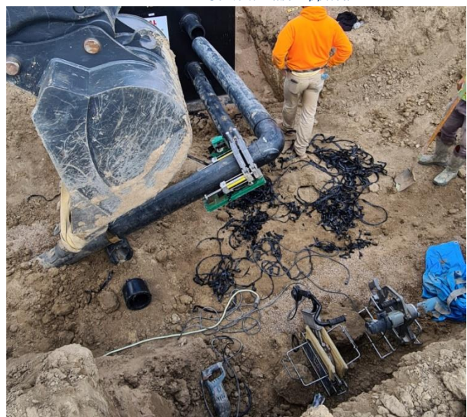
Figure 29 - Geothermal Vault - Preparation to Fuse 8" Supply/Return Lines
