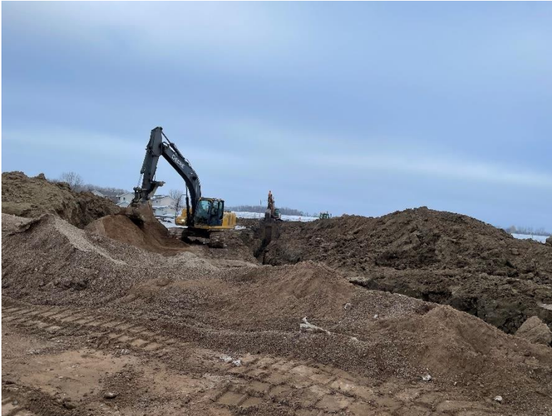
Figure 34 – Trench Excavation for 8" Supply/Return Lines (1/18/2022)
