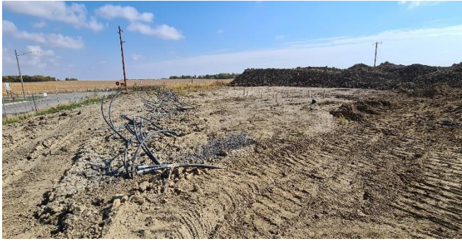
Figure 43 – Loop Ends and Staked Area for Excavation of Trench for Circuit Tie-Ins
