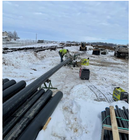
Figure 35 – 8" Pipe Prepared for Fusion
