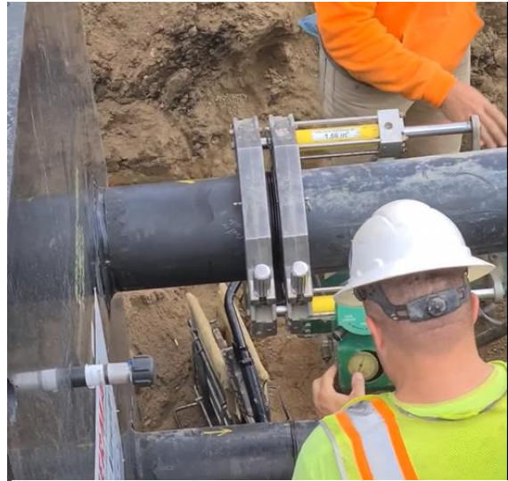
Figure 31 – Checking the Fusion Pressure
