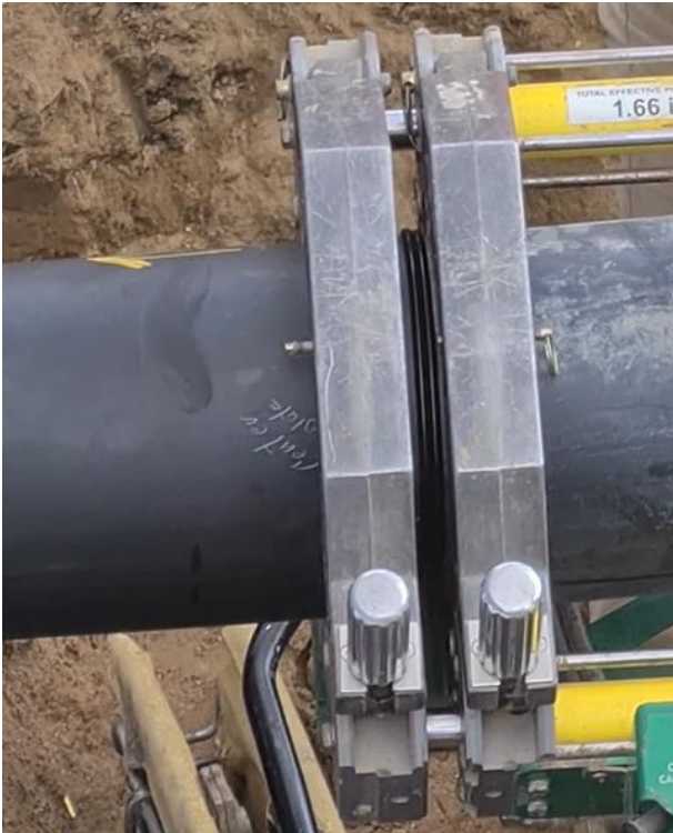
Figure 32 – Supply/Return Fusion of 8" HDPE Pipe
