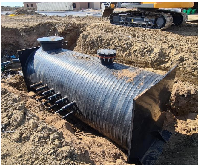
Figure 26 - Geothermal Vault after Placement
