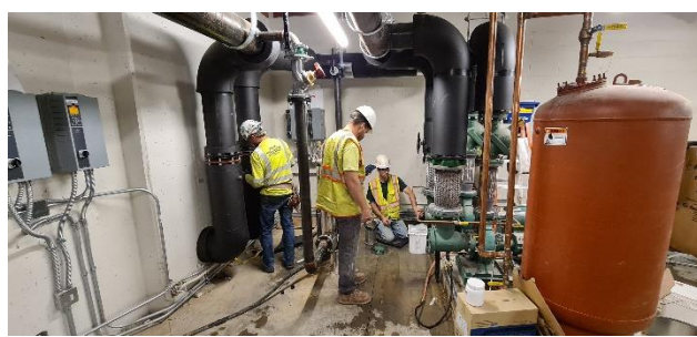
Figure 60 – Preparing the System to Receive Glycol
