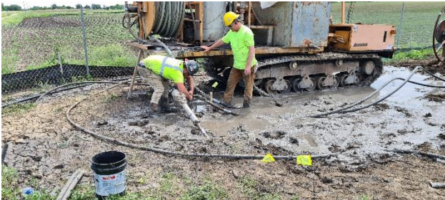
Figure 17 - Preparing to Pull the Loop and Tremie Pipe back into the Borehole
