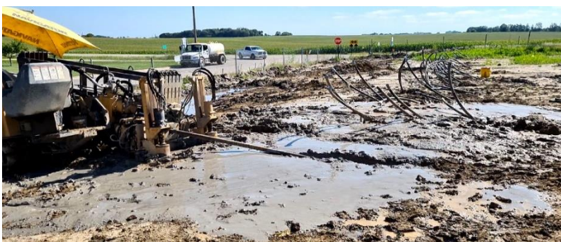
Figure 22 - Loop and Tremie Being Pulled Back Through Borehole
