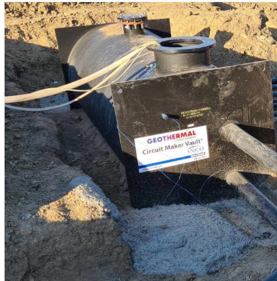
Figure 27 - Geothermal Vault After Cement Base Applied
