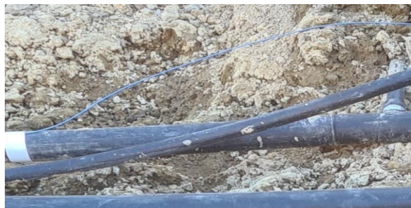
Figure 49 – Tracer Wire on Each Circuit
