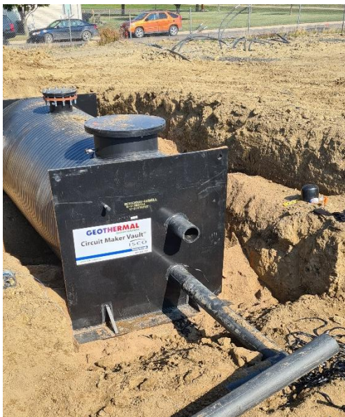
Figure 28 – The First 8" Supply/Return Line is Fused to the Vault
