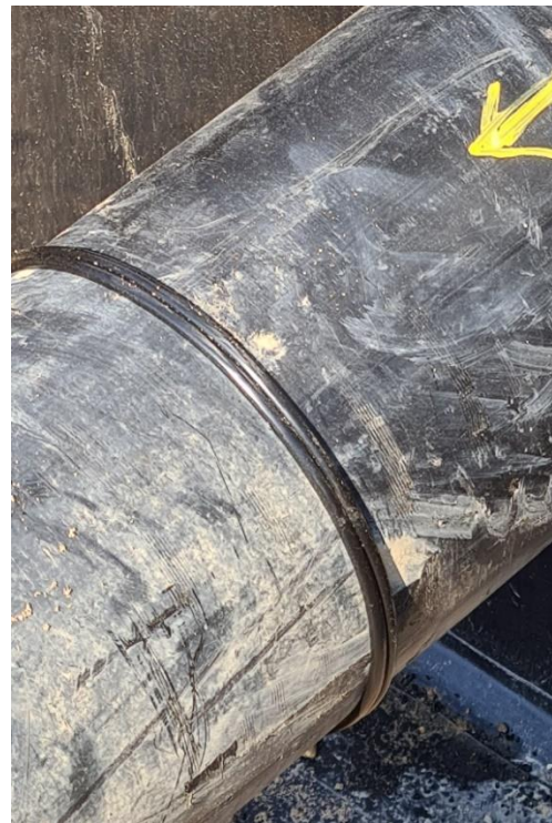
Figure 33 – Supply/Return Fusion of 8" HDPE Pipe
