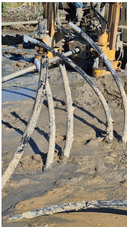
Figure 21 - A Row of Loops After Grouting
