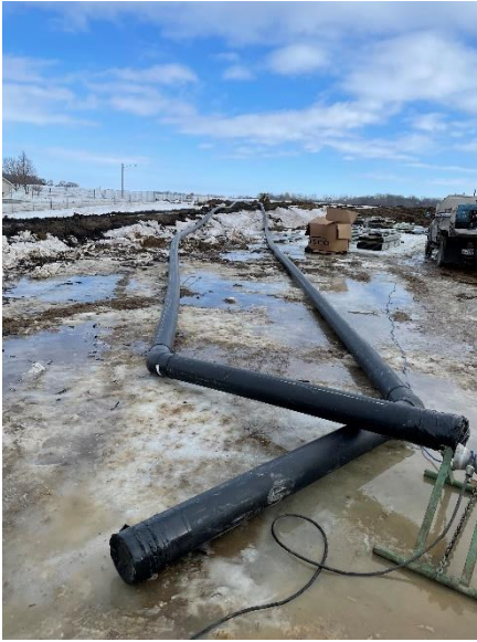
Figure 38 – Pre-fused 8" Lines Ready to be Placed in Trench Between Building and Vault
