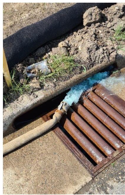
Figure 63 – Evidence of Glycol in System
