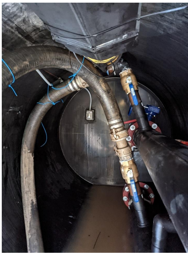
Figure 58 – Interior Geothermal Purging and Filling Connections
