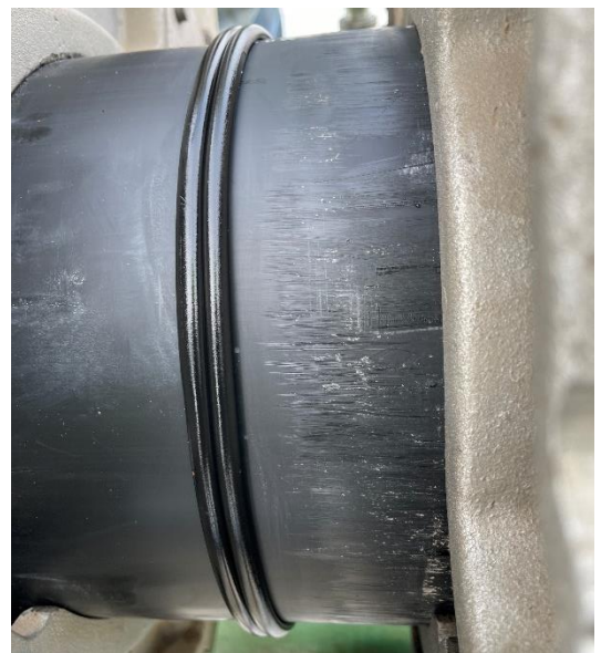
Figure 37 – Completed 8" Fusion Joint
