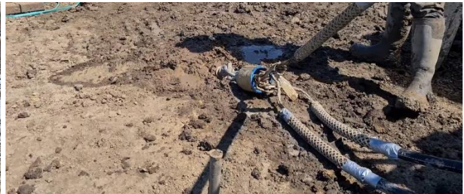
Figure 18 - The Tremie Line and Loop Ready to Pull Back Into Borehole
