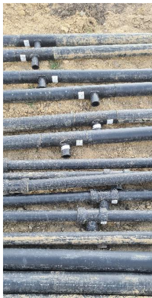
Figure 45 – Factory Tees and Pipe Fusions for Tie-Ins
