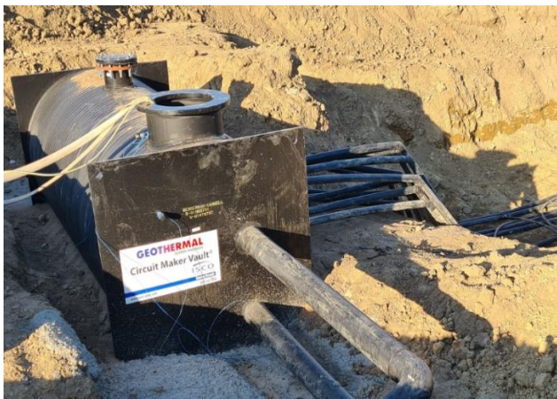
Figure 50 – Circuit Connections from Trench to Vault
