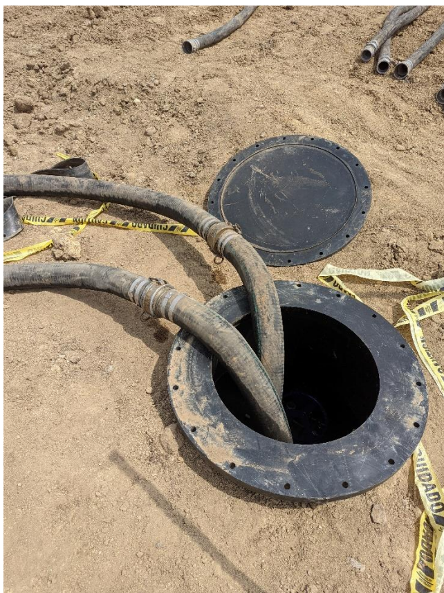
Figure 57 – Pump Connections into Geothermal Vault
