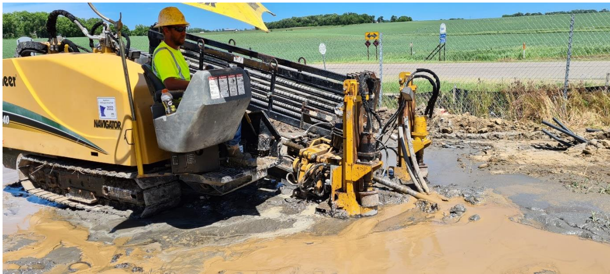
Figure 10 - Vermeer D24x40 Horizontal Boring Machine. Licensed for 2022.
