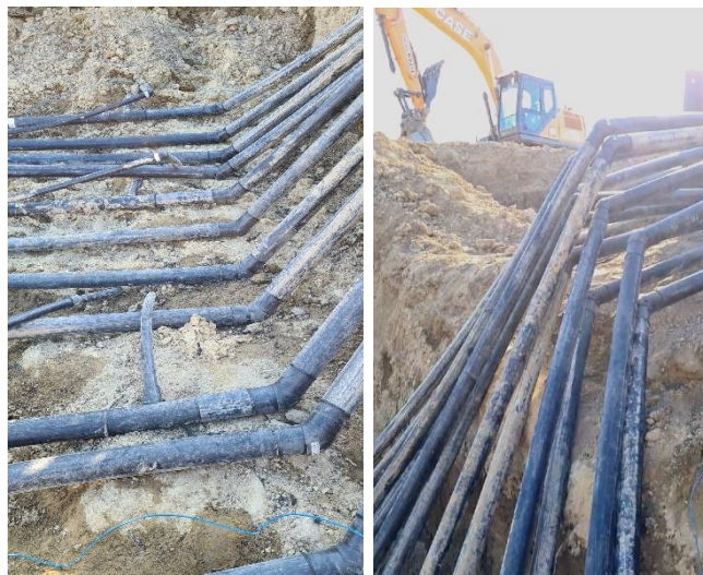
Figure 51 – 3" HDPE Circuits from Trench to Vault Level
