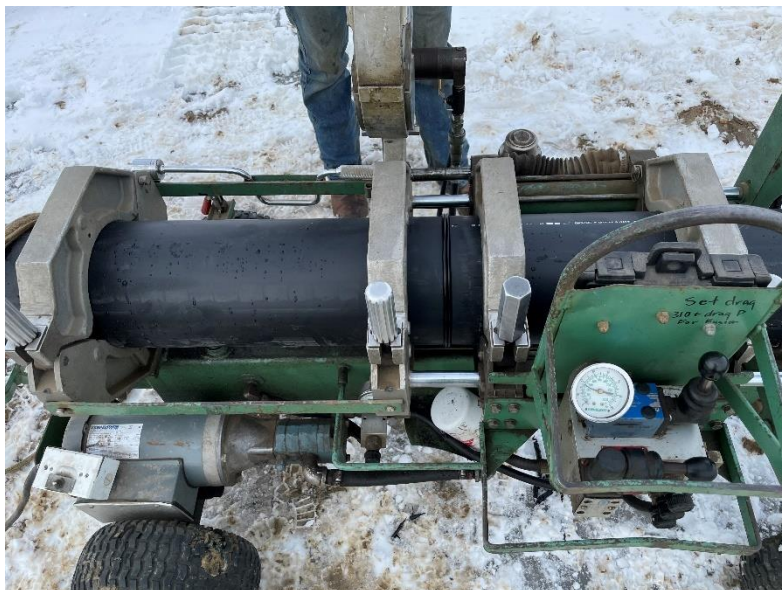
Figure 36 – Fusion Process for 8" Line
