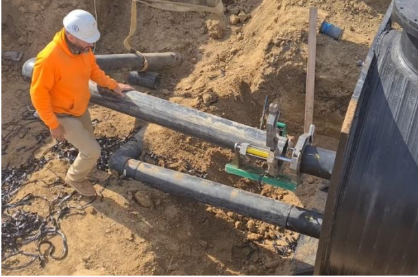
Figure 30 - Fusion Preparation for the 8" Return Line to the Geothermal Vault
