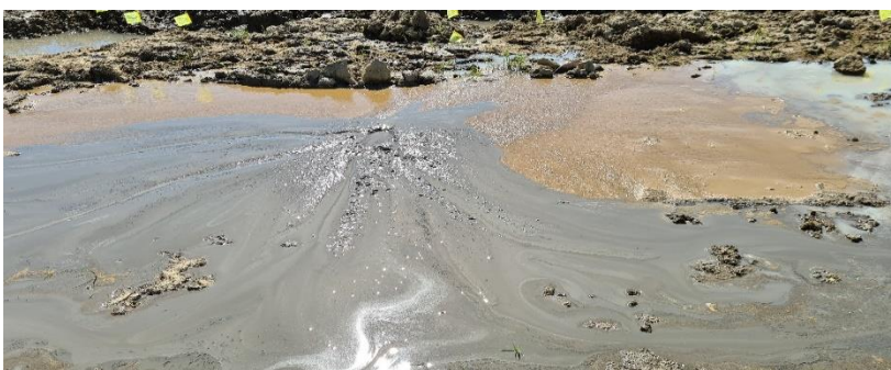
Figure 23 - Evidence of Graphite as Grout is Pumped Into Borehole from Tremie Pipe
