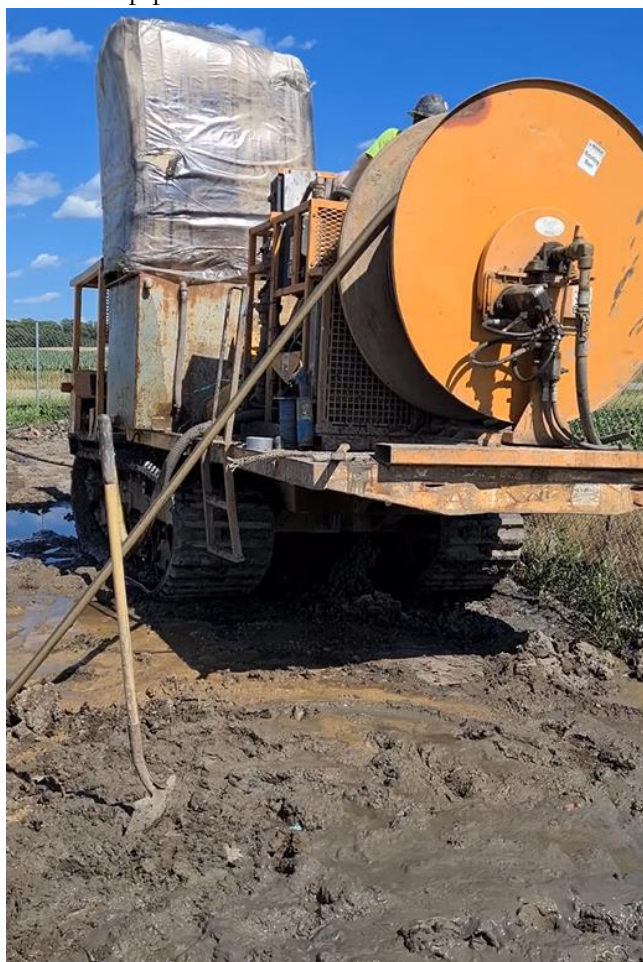
Figure 19 - Grouting Machine and Operator Extracting Tremie Pipe Using a Hydraulic Reel. Note Proximity to Fence.
