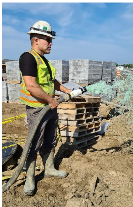
Figure 61 – Flushing the Delivery Line
